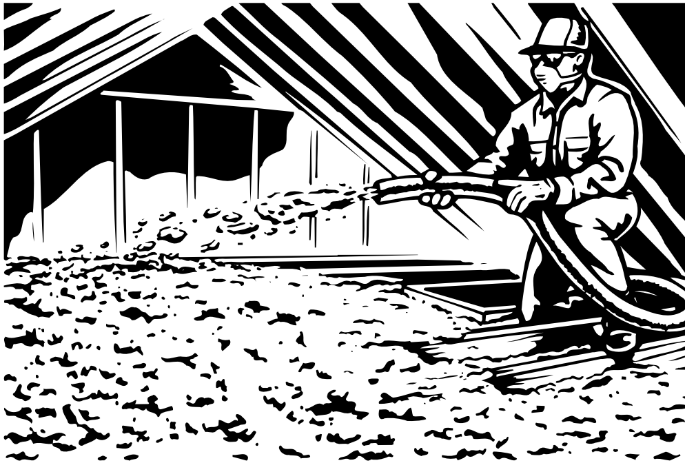
Figure 5. Loose-fill insulation installation
